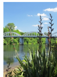
Fairfield Bridge C.GRC.WAI.22
